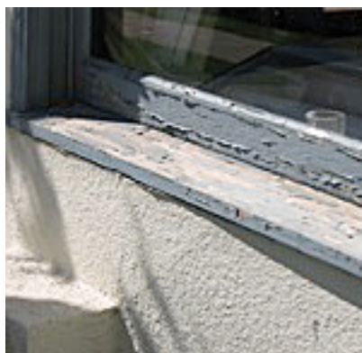
FIGURE 5.4a Peeling paint
