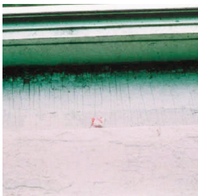
FIGURE 5.4b Alligatoring paint
